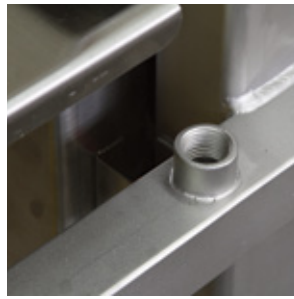
Frame clean-out flushing port.
