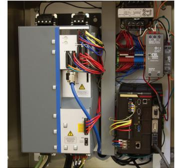
**Custom Controller.** Built-in system/user interface provides up-to-the-minute machine status, history, and diagnostics.
